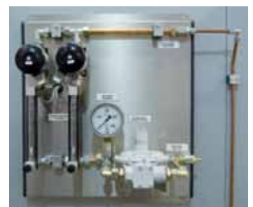
System zasilania gazem do pieca HFL 160/17
